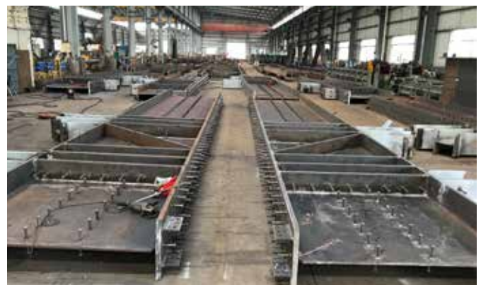
鋼板梁製造 Steel Plate Girder Fabrication
