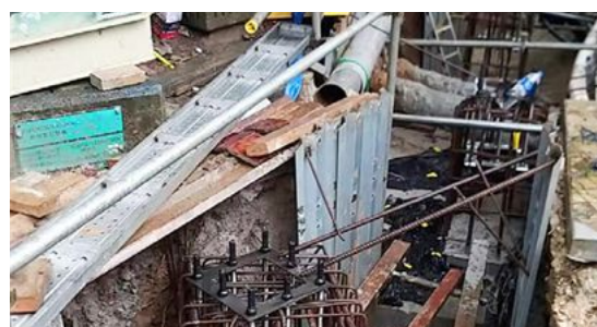
為深度超過1.2米的挖掘溝槽提供支撐設施 Shoring support to excavation with depth greater than 1.2m
