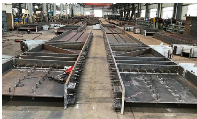
鋼板梁製造 Steel Plate Girder Fabrication
