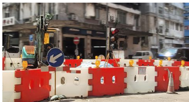
為行車道上的工程採取臨時交通安排 Temporary traffic arrangement for work carried out on carriageway
