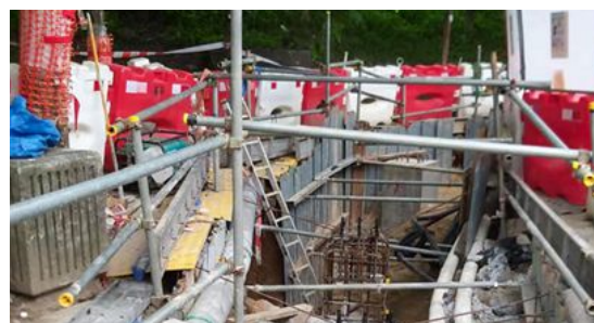
在地下安裝支柱 Support the existing utilities by propping from underneath
